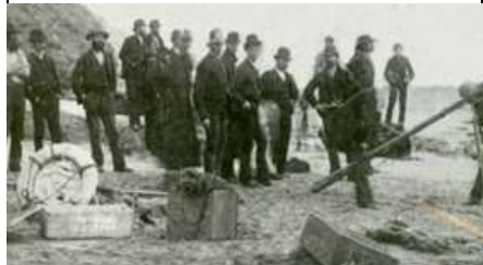
The Rocket Rescue Crew attend the ‘Fiji’, 1891
