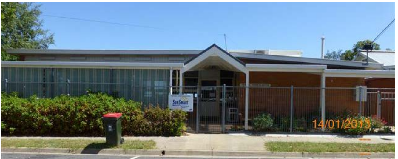
Figure 1: Former Terang Kindergarten, 8 The Promenade, Terang
