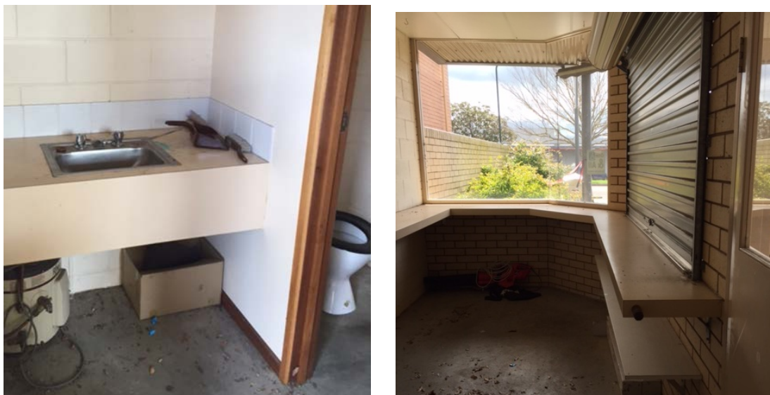
Figure 3 & 4: Internal Photo of 19F Curdie Street, Cobden
