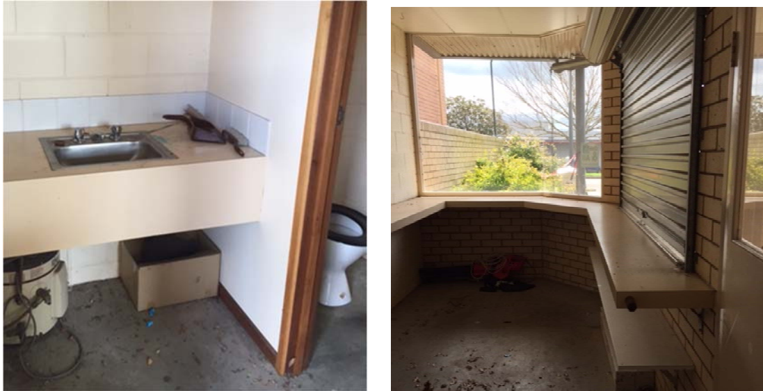
Figure 3 & 4: Internal Photo of 19F Curdie Street, Cobden
