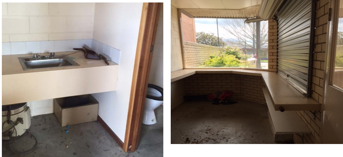
Figure 3 & 4: Internal Photo of 19F Curdie Street, Cobden
