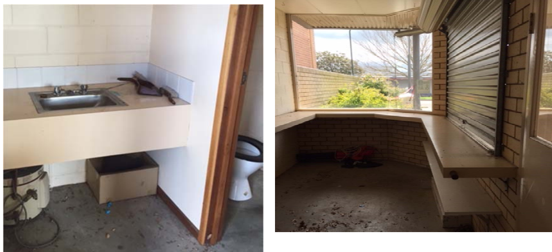
Figure 3 & 4: Internal Photo of 19F Curdie Street, Cobden
