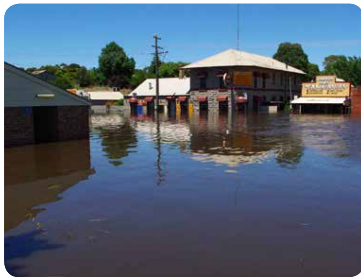
Skipton Hotel, January 2011 flood. Photo courtesy of Corangamite Shire Council.
