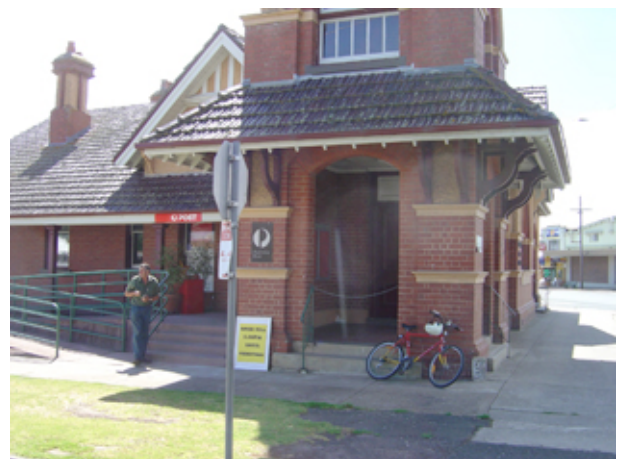
The installation of bike parking rails is recommended for a number of locations in the town – such as the Post Office.
