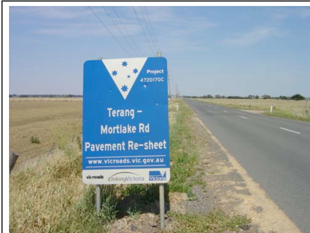
Pavement re-sheet on Terang Mortlake Rd. 3.8m wide lanes; edge line could be at 3.2, with 0.6m wide shoulder.
