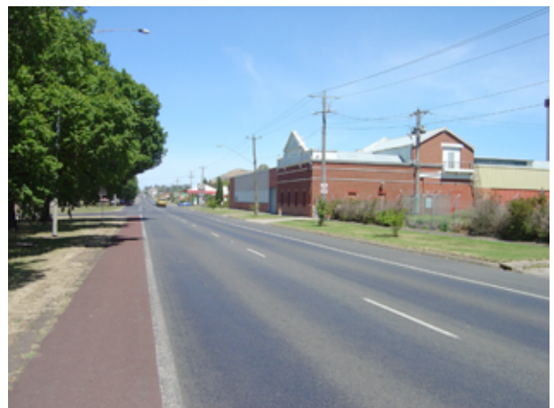
The use of red coloured asphalt on the shoulders of Princes Hwy is an excellent technique for distinguishing on-road cycling facilities.
