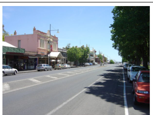
Though bike lanes exist along Princes Hwy through Camperdown, the lane lines are faded and logos are difficult to find.
