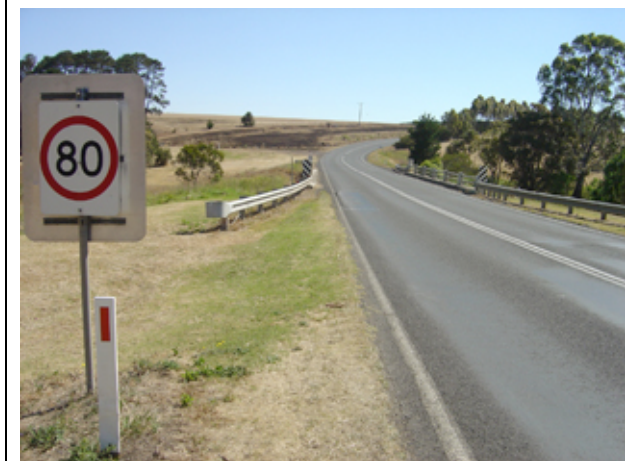
Consideration should be given to the relocation of the speed zone sign to the east of the bridge.
