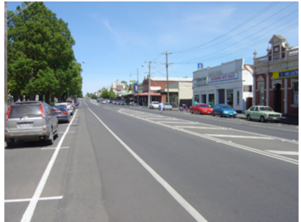
In some locations the bike lane lines on Princes Hwy through Camperdown are very visible, though the addition of logos is recommended.
