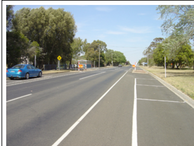
Bike lanes have been installed on McKinnons Bridge – Noorat Rd outside the Noorat School.
