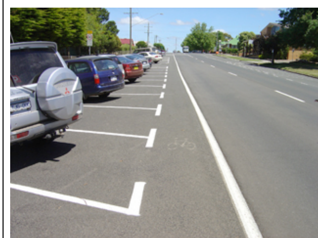
Throughout Cobden is evidence of previous work to identify an on-road cycle network. Faded bike lane logos should be re-instated.
