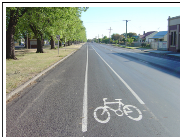
Bike lanes have already been installed on the Camperdown Lismore Rd, between Princes Hwy (Manifold St) and the railway.
