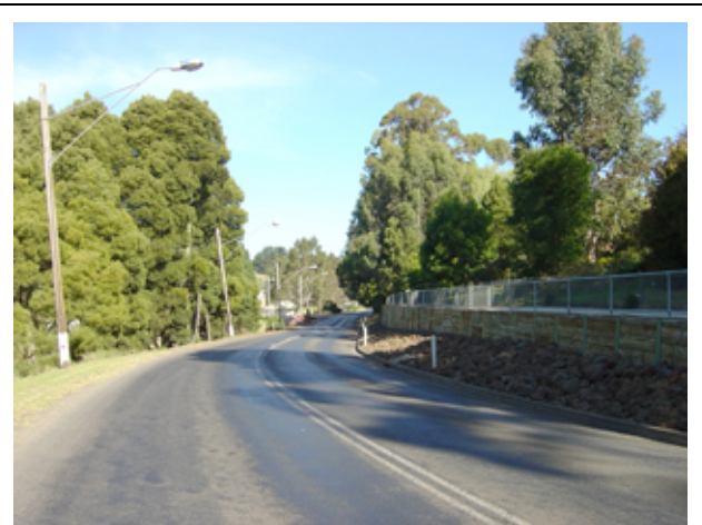
Where the lane widths along Bailey St become narrow, localised road widening to create a sealed shoulder is recommended.
