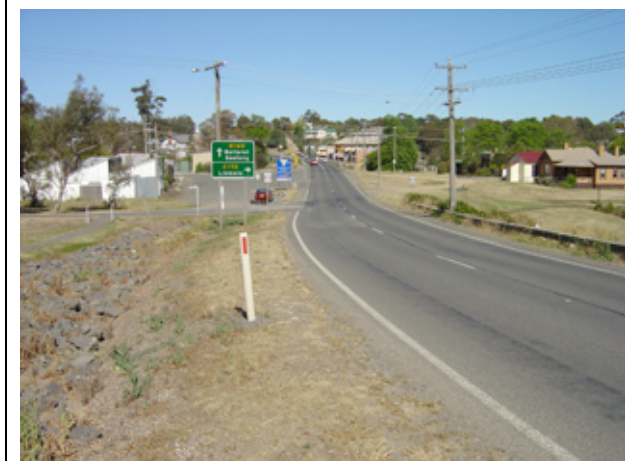
The shoulders of the Glenelg Hwy on the western outskirts of town should be widened and sealed to accommodate cyclists.
