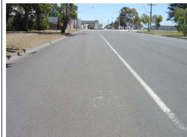
The shared parking and bicycle lane lines and logos on Curdie St need re-painting.
