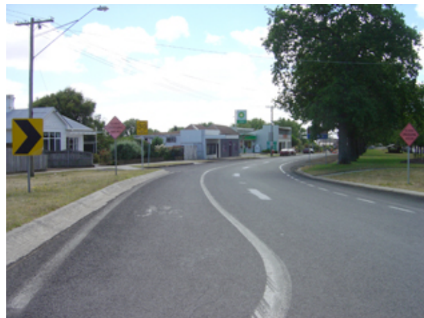
Marked bike lanes occur on Princes Hwy through Terang. However, lane lines and logos are fading and need re-marking.
