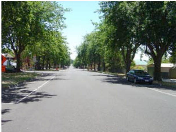
Some local streets such as Brooke St are important links in the cycle network, and are wide enough to have marked bike lanes.
