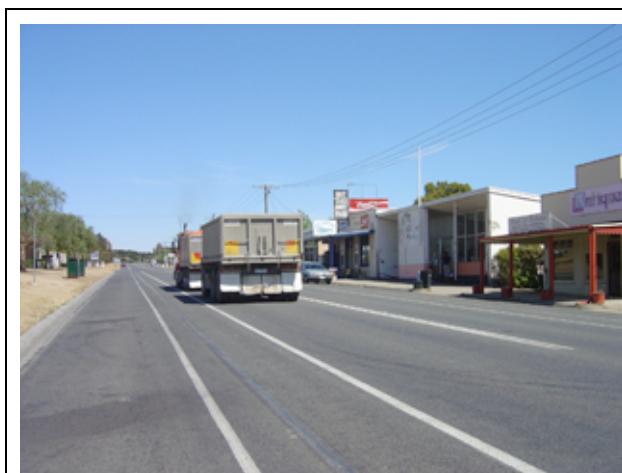
Hamilton Hwy through Lismore carries heavy haulage traffic. Bike lanes do exist, as a result of reducing traffic lane widths.
