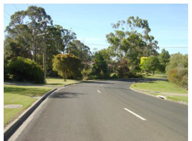
Curdievale Road in Timboon is wide enough at 4.6m in each direction for a 1.5m bike lane both sides.
