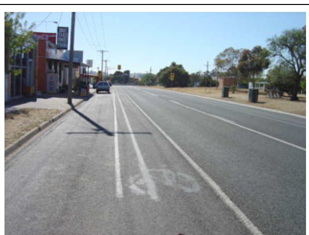
The logos in the bike lanes along the Hamilton Hwy in Lismore appear to have been decommissioned.
