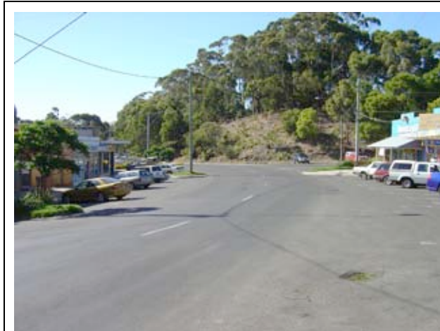
The main road through Timboon has adequate width to accommodate marked bike lanes.
