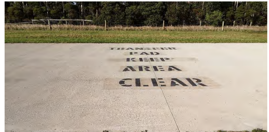
Figure 8 Helicopter transfer pad
