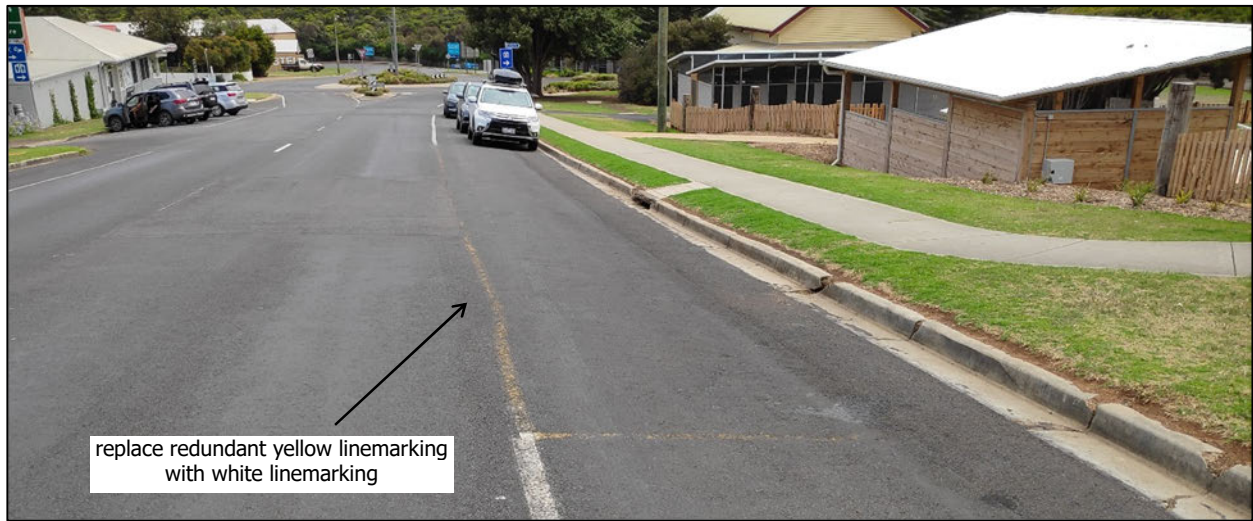
Figure 3.12 Morris Street Parking at New Public Toilets (ID-6a)
