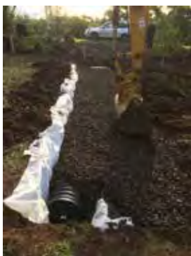
Alternative waste water system on constrained site
