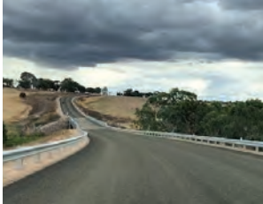
Roads, footpaths & drainage
