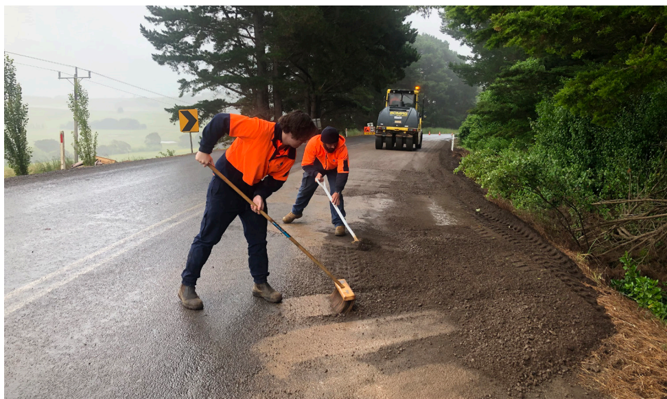
Works teams continue to improve roads across Corangamite Shire
