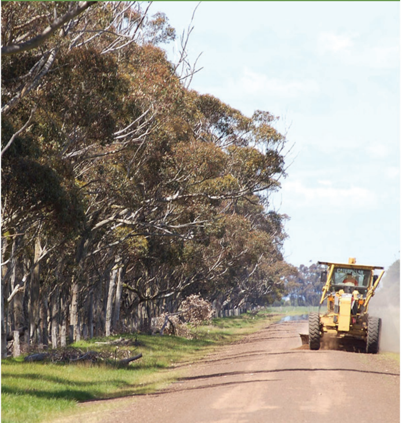
Routine Road Maintenance
