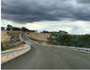
Roads, footpaths & drainage
